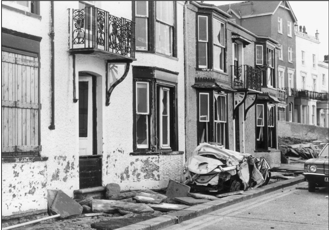
Figure 5.3 – Damage at Herne Bay as a result of 1978 Storm
