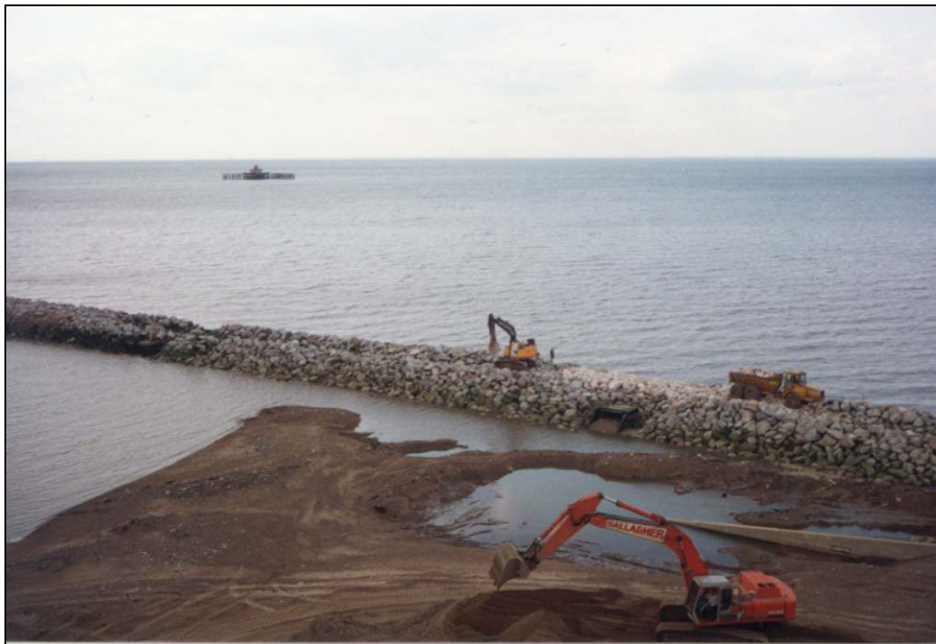
Figure 8.1 – New sea defences under construction at Herne Bay in 1990
