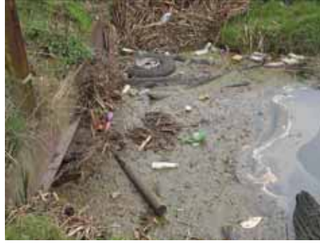
Blockage causing sluggish flow and siltation problems
