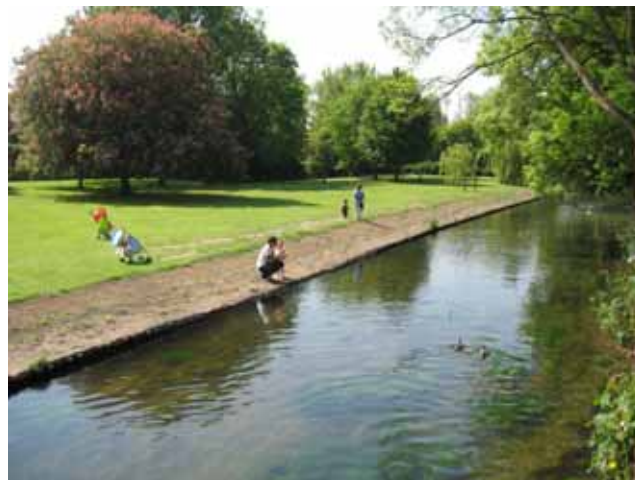
Timber edge removed and bank regraded
