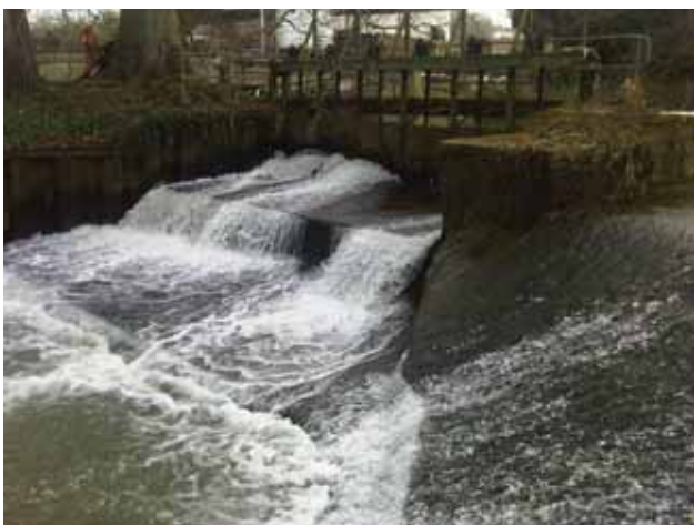
Weir upstream of Chartham Paper Mill
