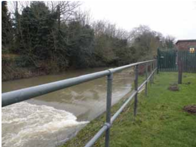
Environment Agency flow gauging weir
