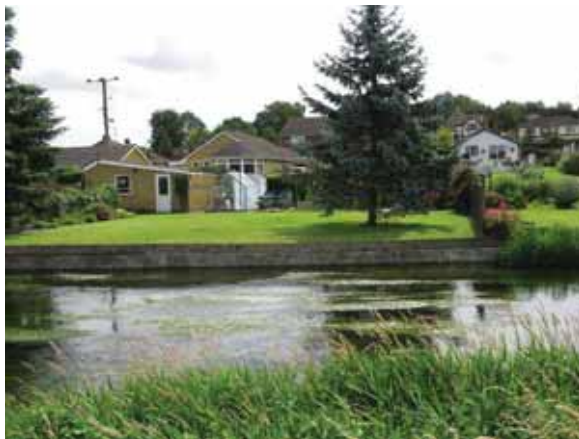
Hard revetments close to Tonford Bridge
