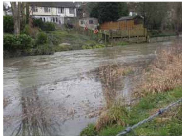
Natural Berm – A complimentary berm on the opposite bank would create a pinch point of fast water.
