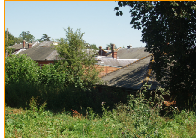
Figure 8 Example of building levels in the west of the site and the buildings cut into the slope
