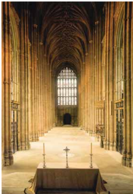
The Nave looking West
