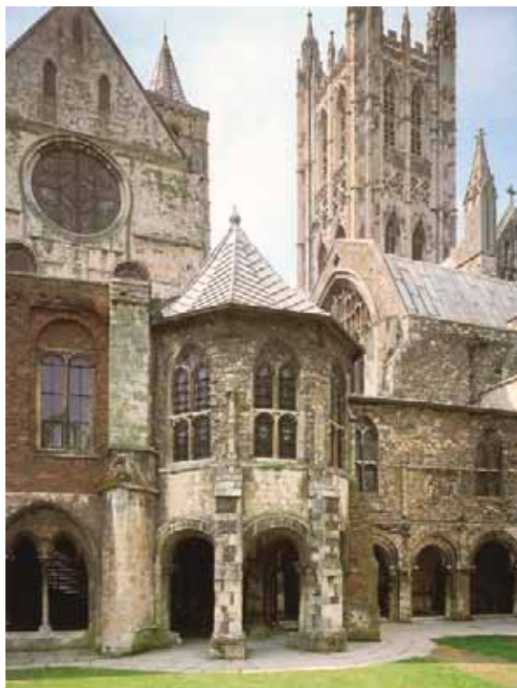
Prior Wibert's Water Tower
