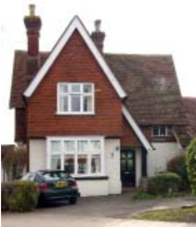
28 South Canterbury Road
