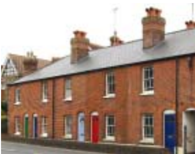
Below: 102 to 120 Old Dover Road.
