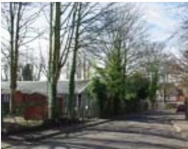
Below from top: Old Ruttington Lane, Clyde Street/Alma Street, 57 to 61 Military Road (Dairy Crest).
