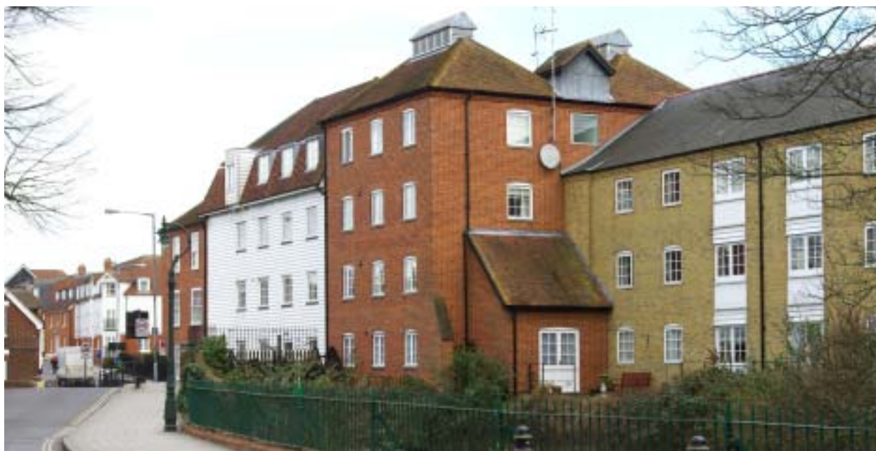
Deans Mill Court
