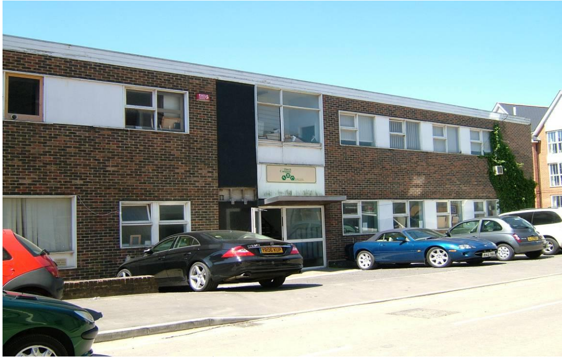
View of part of site showing office buildings
