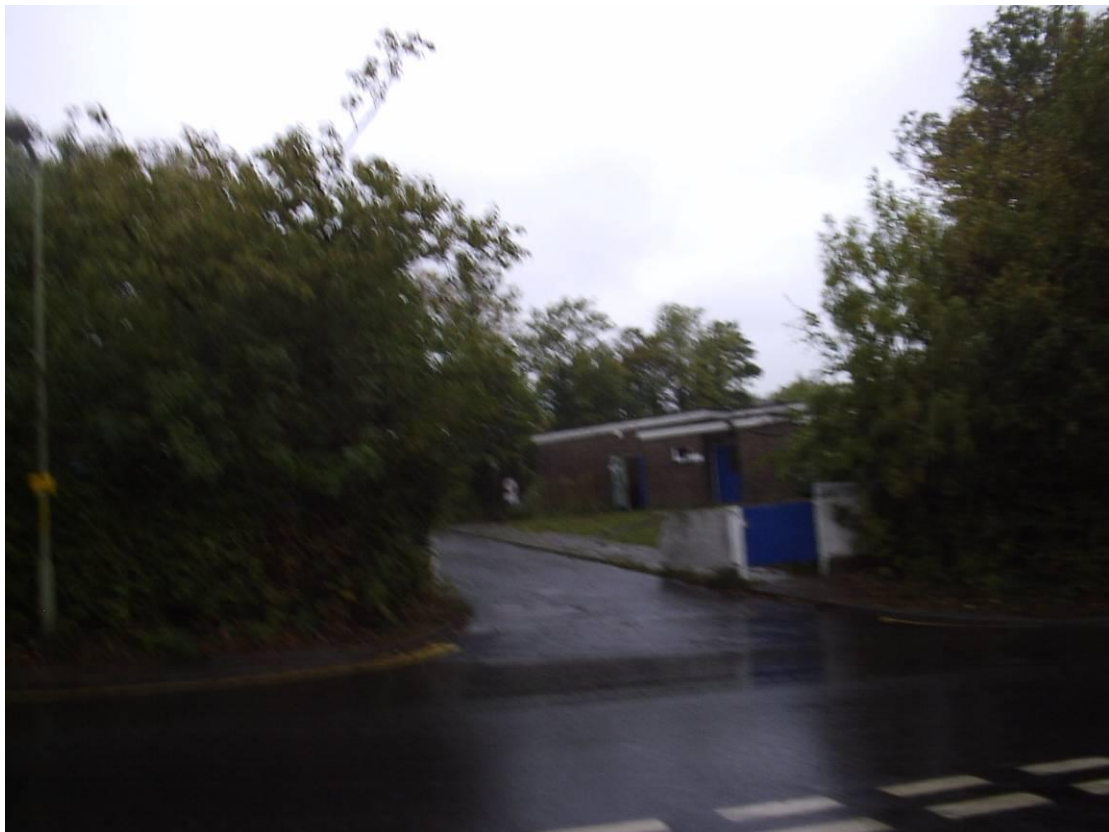
view of site entrance
