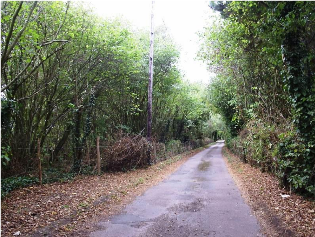
Access way at Alcroft Grange
