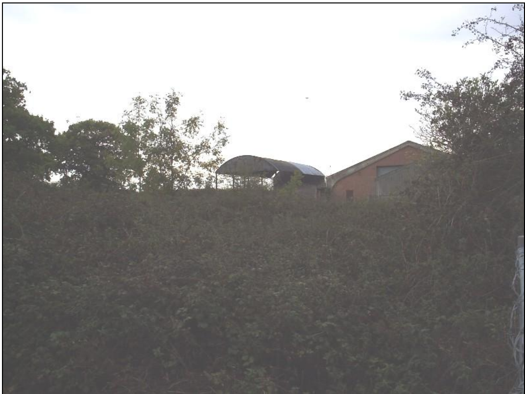
Existing buildings on site
