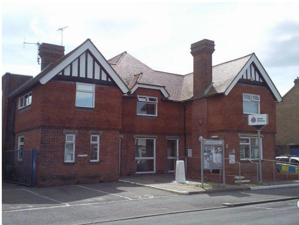
Photograph of front of site
