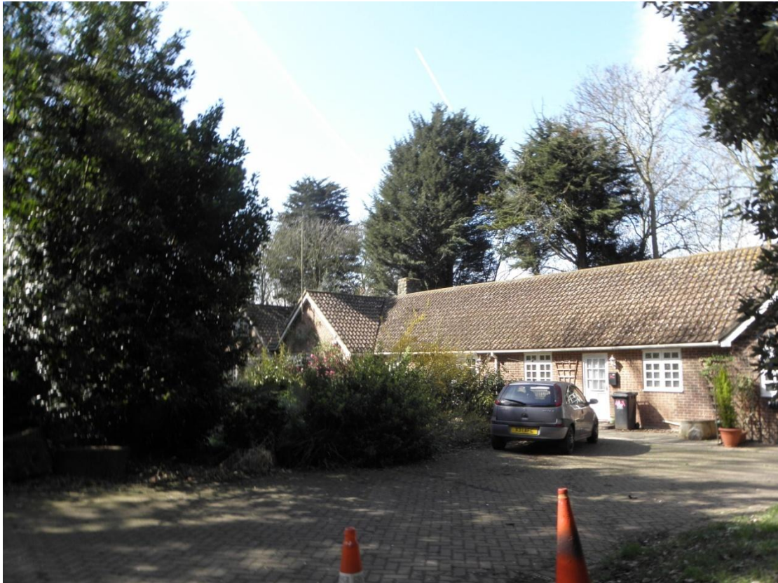
View of terraced bungalows
