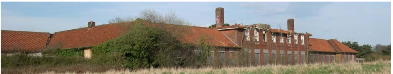
Oak House – the main complex
