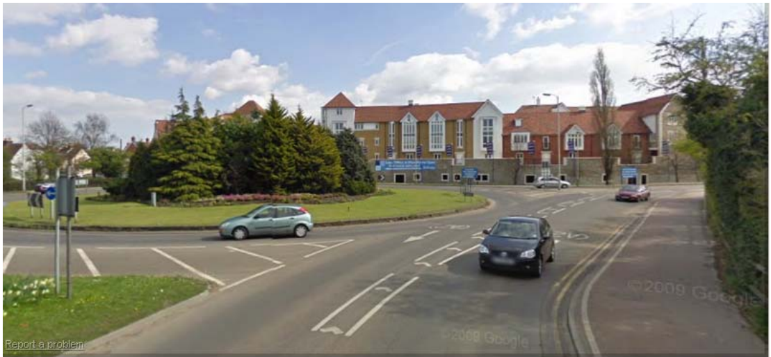
Figure 4-3 Example of detailed photograph used for junction modelling. Source: Google Maps ©2010Google
