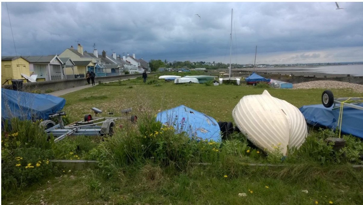
Looking south along beach towards the Caravan Park – seawall and beach huts to left
