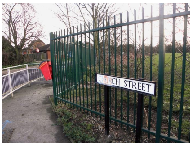
Fence that surrounds site
