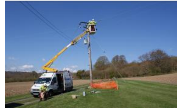
Removing overhead cables
