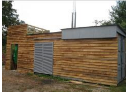
Oak clad woodfuel boiler
