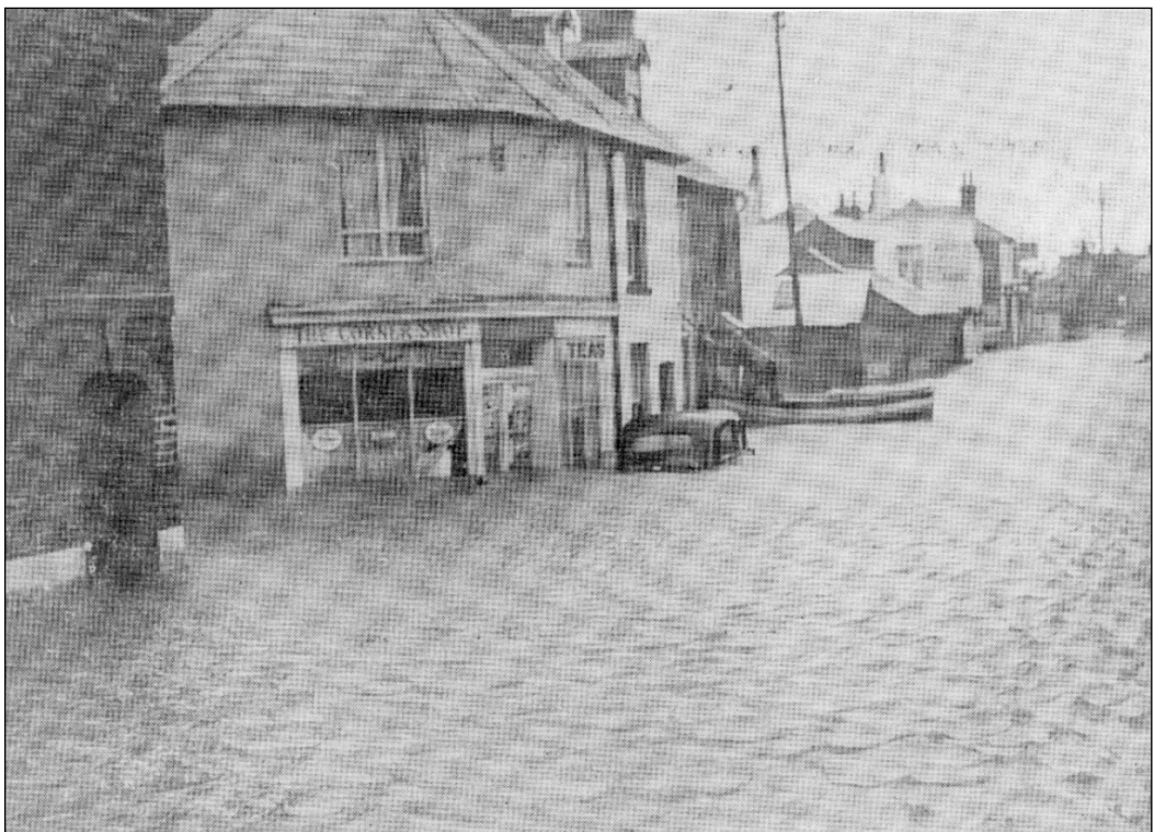
Figure 4.2 - Flooding at Whitstable, January 1953
