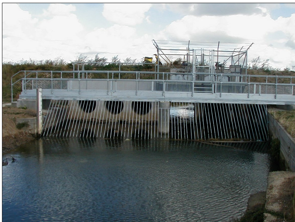
Figure 4.9 - Improvement to the Swalecliffe Brook Outfall
