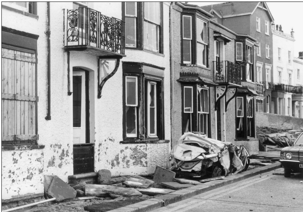
Figure 4.3 - Damage at Herne Bay as a result of the 1978 Storm
