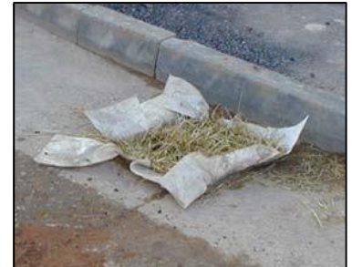
Protected Drain using
