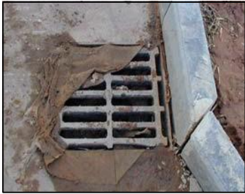
Protected Drain using Terram Straw
