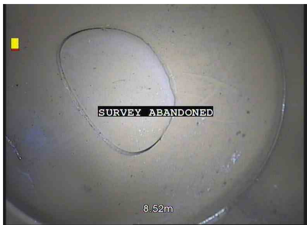
004.jpg, 00:01:48, 8.52 m Survey abandoned, Unable to round bends to rwp
