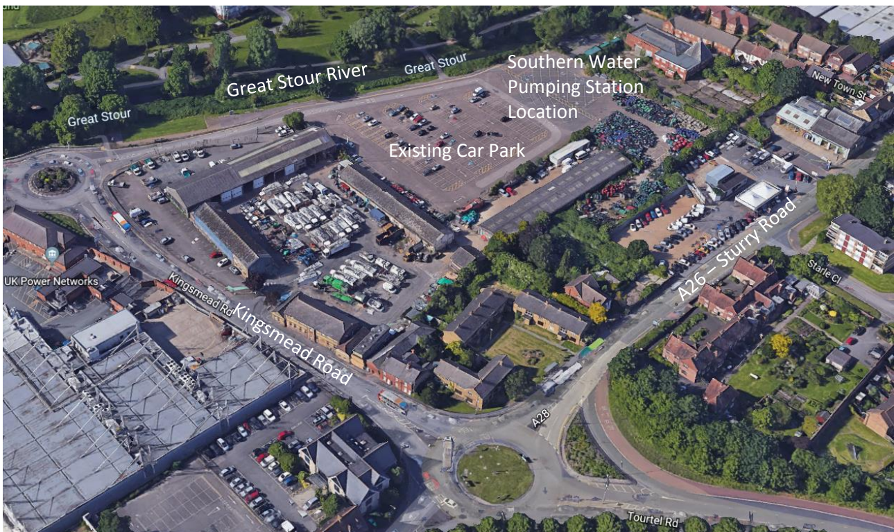
Figure 4 - Aerial View of Canterbury Site Pre-development (Google Maps Capture)
