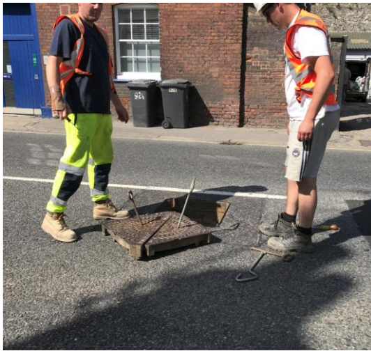
Frame 2 ~ Cover to TR15582001 removed under traffic control
