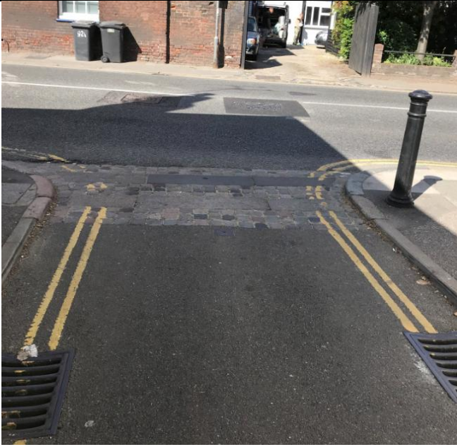
Frame 1 ~ Road Gullies at the end of Old Ruttington Lane looking towards Broad Street
