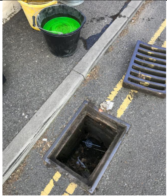
Frame 2 ~ Gully Frame lifted and bucket of water with fluorescent drain dye seen in background ready to pour in the gully
