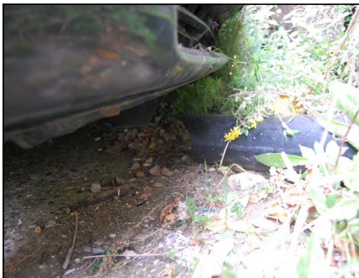
RWP 4 OUTFALLS TO GROUND
