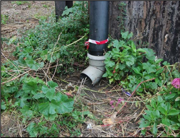
RWP 2 OUTFALLS TO GROUND
