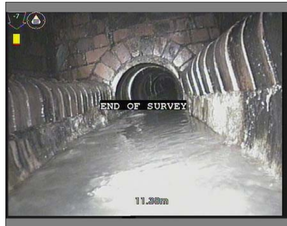
Photo: 002.JPG, VCR No.: 00001 11.38m, Manhole
