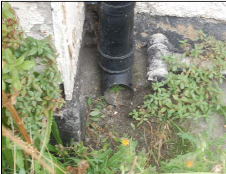
RWP 6 OUTFALLS TO GROUND
