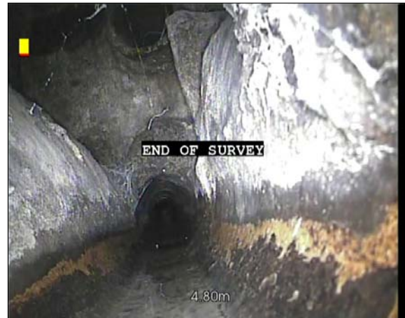
Photo: 019.jpg, VCR No.: 00007 4.8m, Manhole
