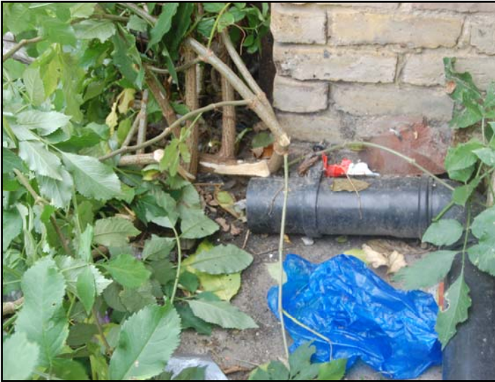
RWP 5 OUTFALLS TO GROUND
