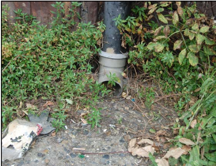
RWP 3 OUTFALLS TO GROUND
