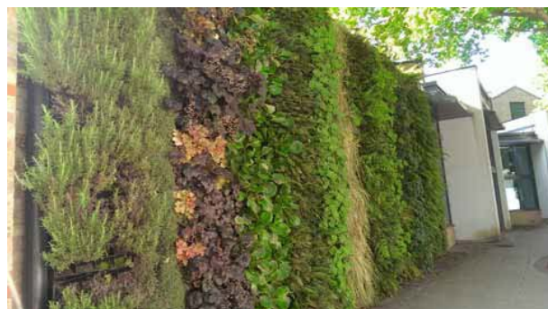
Plate 4.53 Living wall to Aphra Lumley Building
