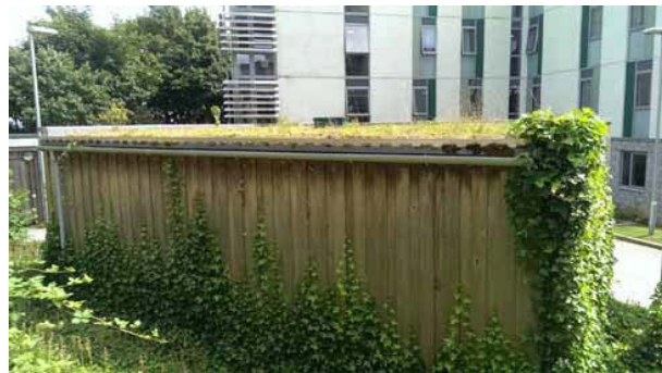
Plate 4.52 Sedum roof to Turing College Store
