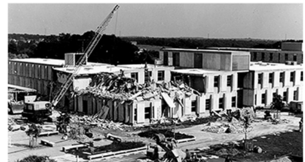
Cornwallis Building - collapse due to railway tunnel, 1974.
