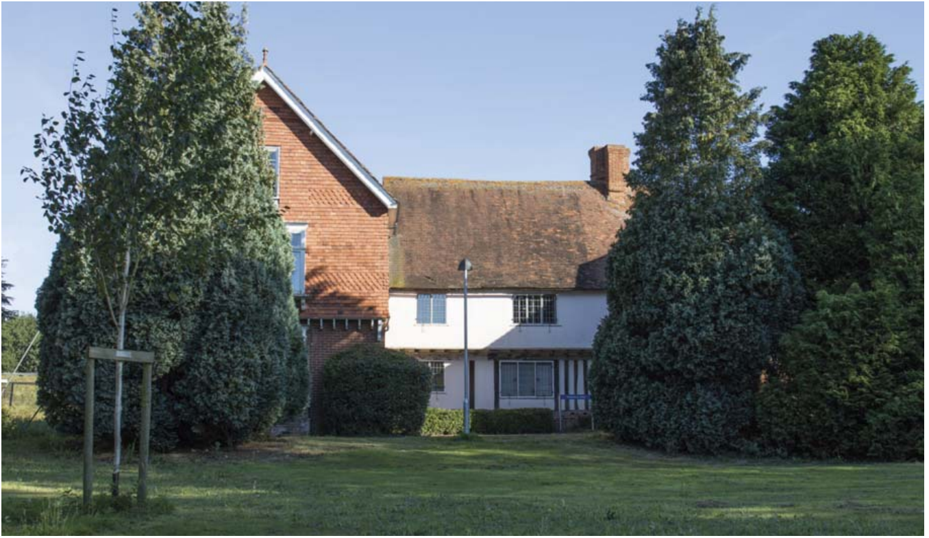
Figure 42: Originating from the 15th century, Beverley Farmhouse is a Grade II listed building
