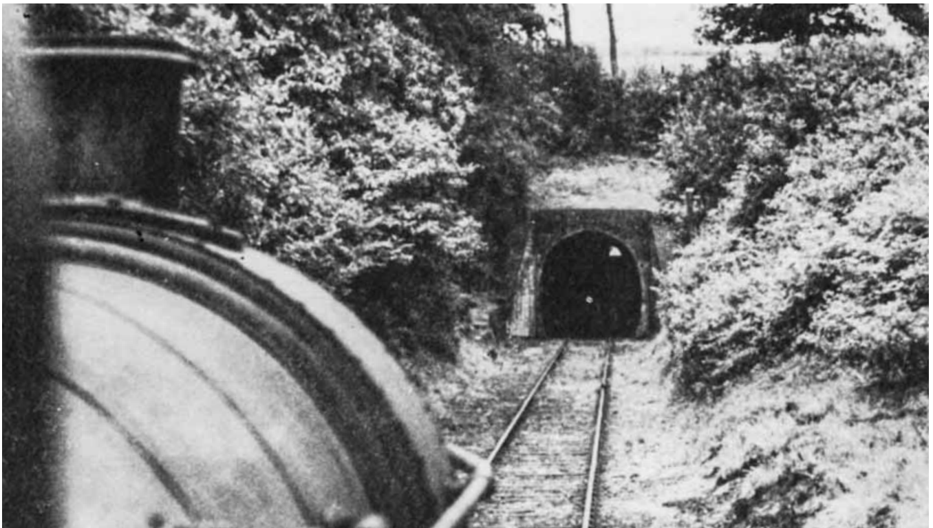
Figure 49: Views of the former Crab and Winkle railway and the North Portal of the Tyler Hill Tunnel
