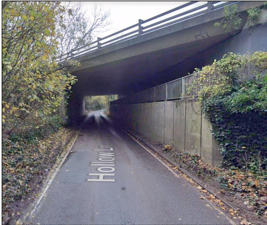
Figure 4.1: Existing Hollow Lane Underpass (Street View)
