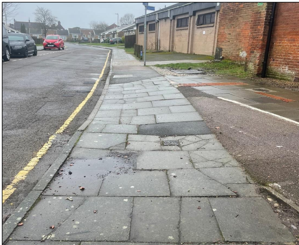
Figure 3.9: Footpath to Rear of Barracks
