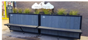
SuDS planter takes water from downpipe/library roof
