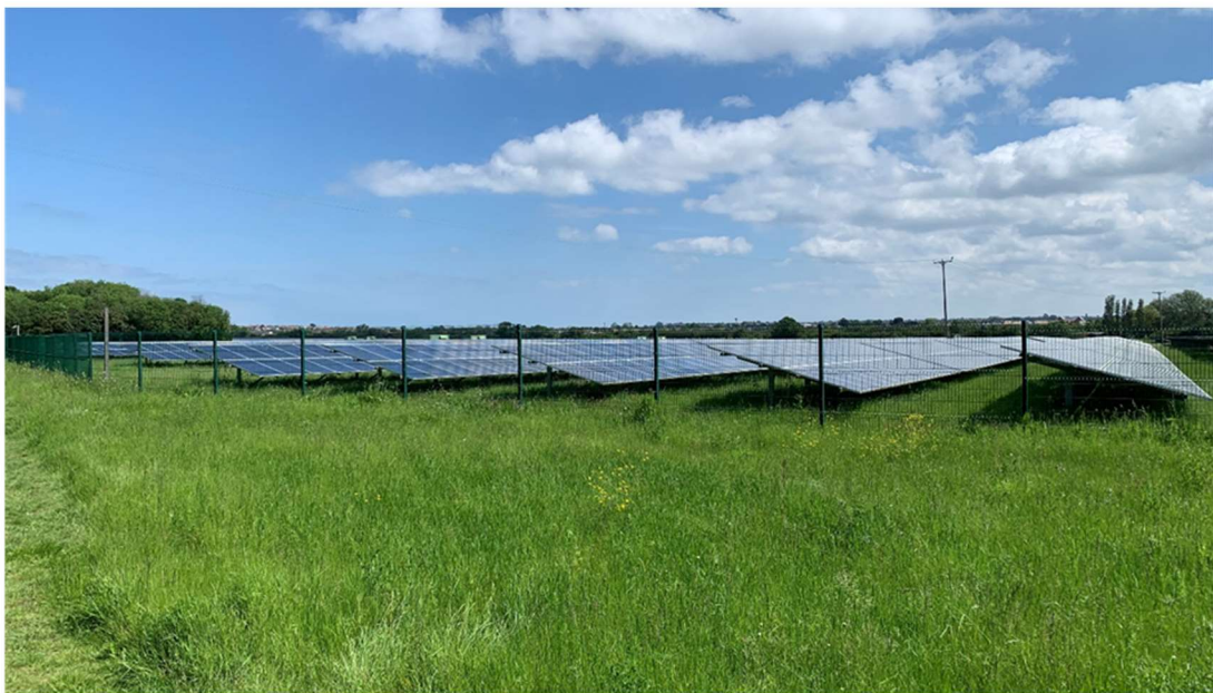
Plate V: Red House Farm Solar Farm is prominent in views from footpaths in the Green Gap, as well as Molehill Road
