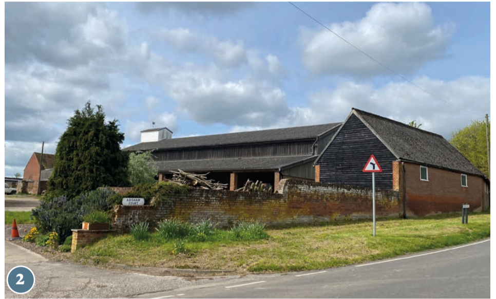
2 Adisham Court Farm agricultural buildings.
