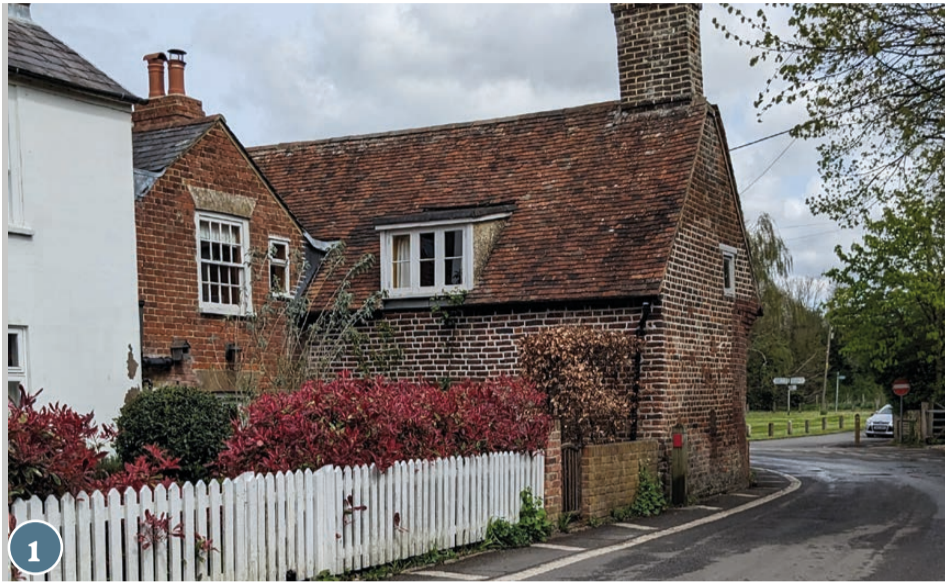
1 Historic buildings on The Street.
