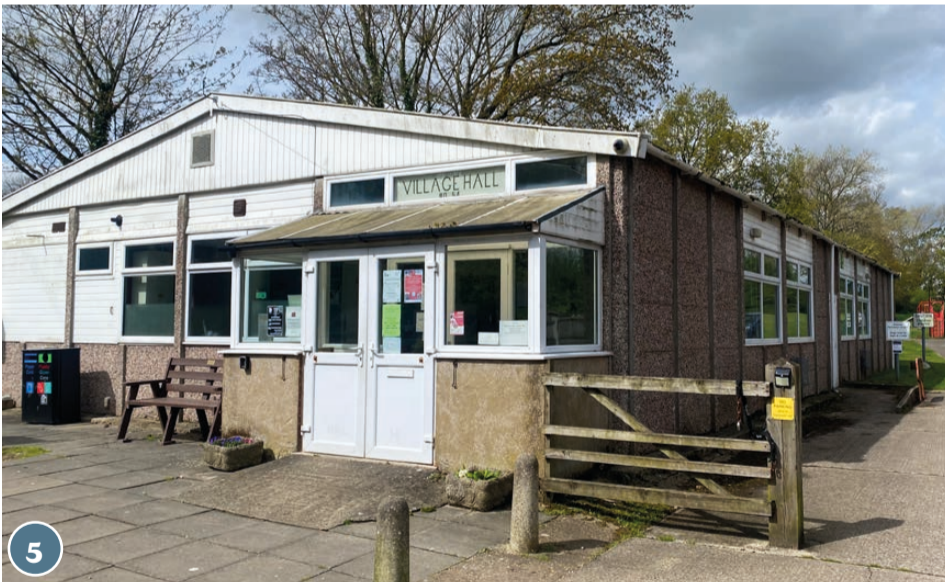
5 Adisham Village Hall.
