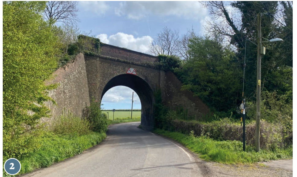
2 Station Road passes under the rail bridge.
