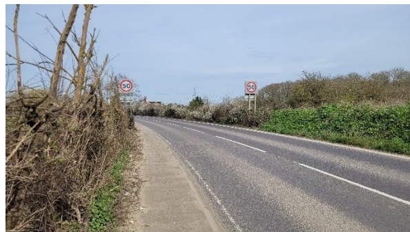
Photo 2 - Herne Bay Road looking north
