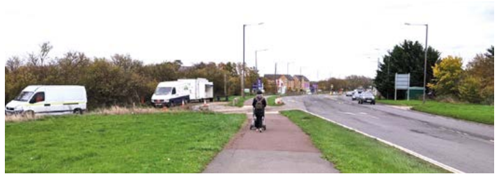
Garden Towns such as Taunton, Bicester and Aylesbury are to expand by building new estates along new sections of ring road around the outskirts of the town like this one we saw on our visits. This ring road model of development divides communities as much as connecting them.
