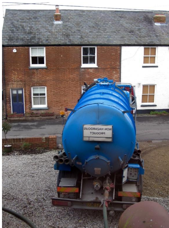
Figure 4 Tankering from Nargate Street, Littlebourne
