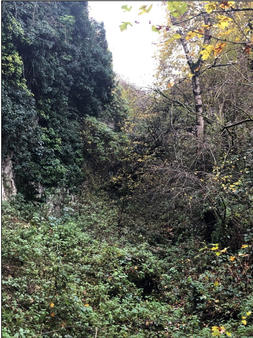
PLATE 11 – UNACCESSIBLE AREA OF VERTICAL CLIFF EXPOSURE
