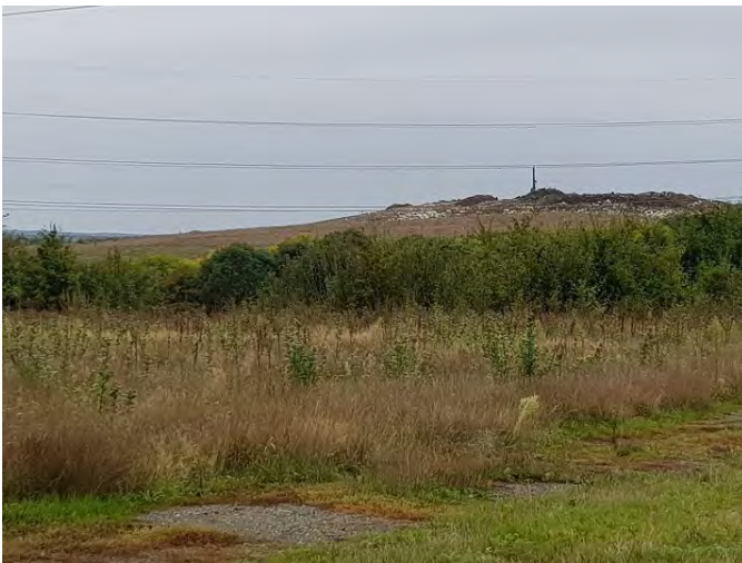
Shelford landfill and gas recovery
