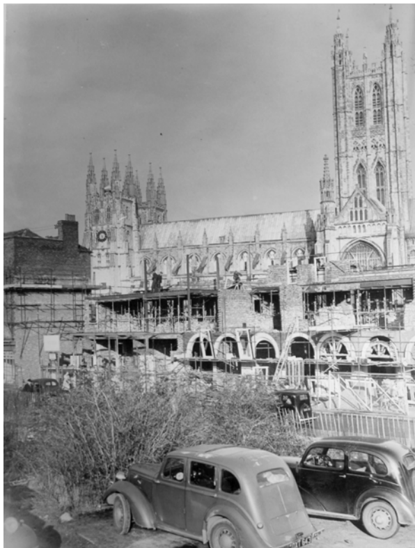
A photograph showing new buildings under development in Burgate, following Second World War bombing, January 1951 (Canterbury Library and Local Studies: 178, copyright unknown)
