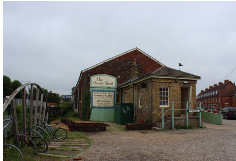
The Goods Shed adjacent to Canterbury West Station
