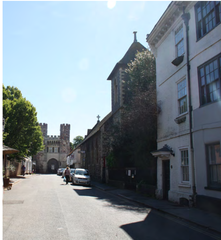
This important local view looks along Church Street St Paul's towards the Cemetery Gate of St Augustine's Abbey with St Paul's Church to the right
