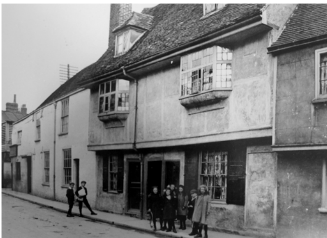
This image shows Stour Street, c.1900, focusing on a refronted medieval building, which retains its jetties. (Canterbury Library and Local Studies)
