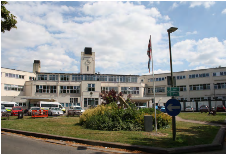
Main Kent and Canterbury Hospital building
