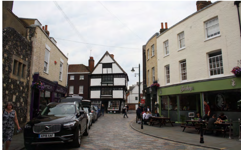
No.28 Palace Street is an example of a timber-framed jettied building within the city, many buildings like those also visible in this picture now bear a polite classical appearance of brick, sash windows and a parapet
