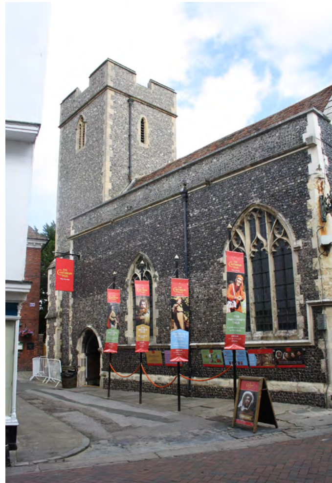
High status buildings such as churches are constructed in stone such as the former St Margaret's Church
