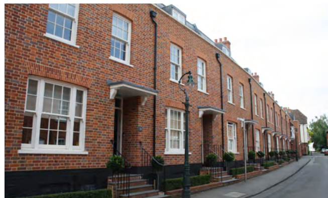
Recent terraced row in St Peter's Lane which is in keeping with the character and appearance of the area
