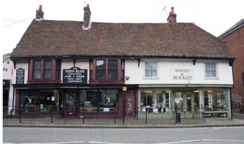
Examples of some of the many shopfronts in the conservation area which exhibit historic and traditional features.
