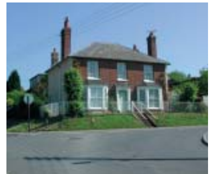
Park House on the corner of Hatch Lane
