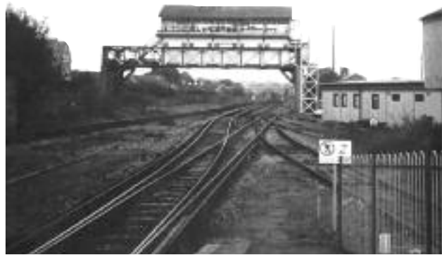
The Signal Box, Canterbury West Station (grade II)
