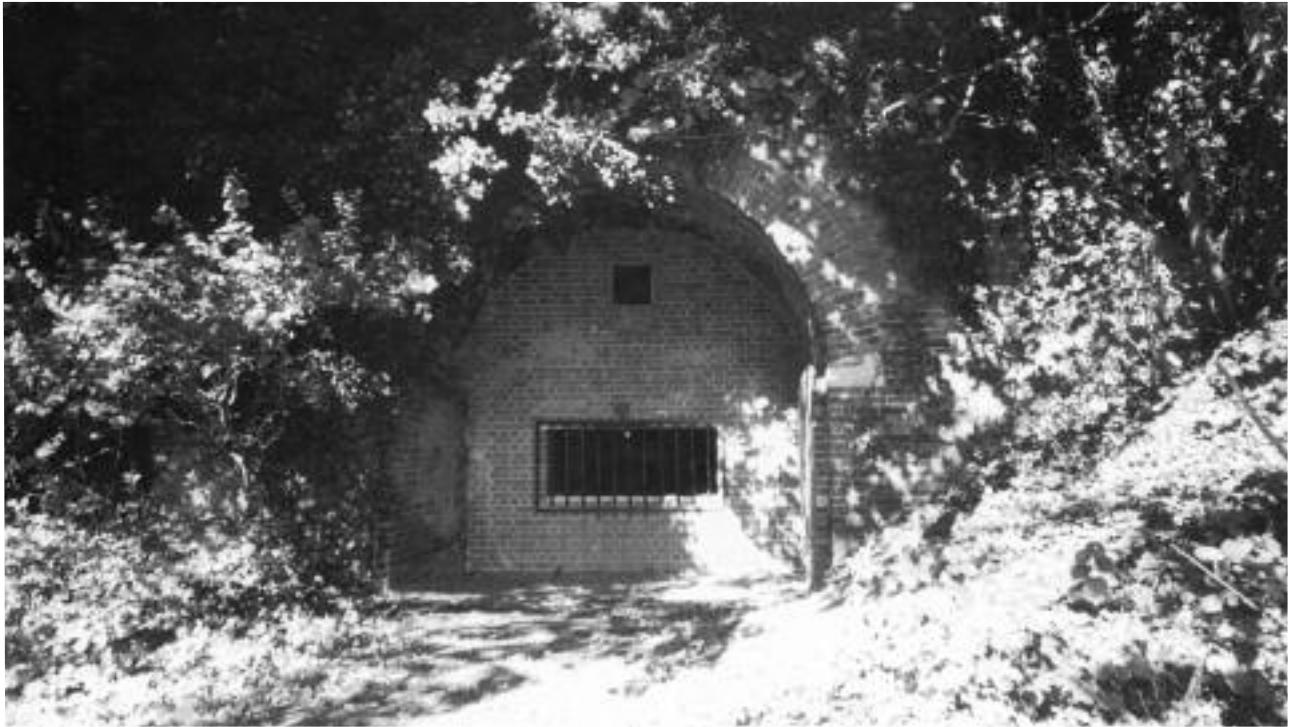
Southern entrance to Tyler Hill Tunnel
