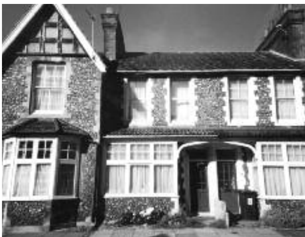
Nos. 11, 13 and 15 Beaconsfield Road
