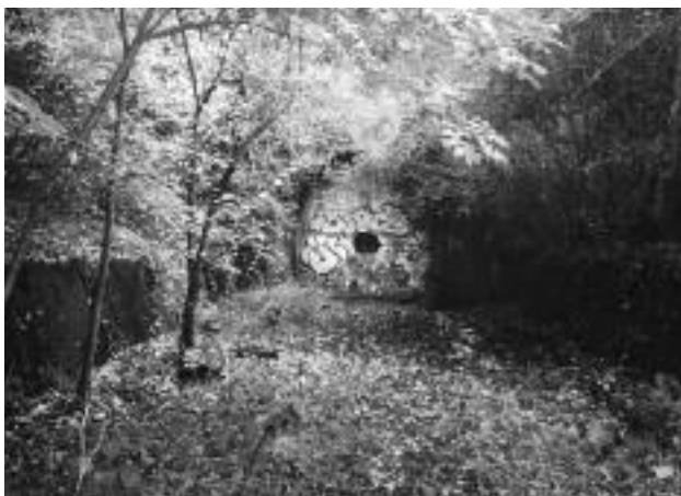
Northern entrance to Tyler Hill Tunnel
