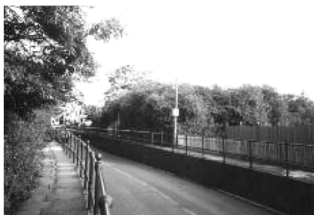
Teynham Road showing site of former railway bridge
