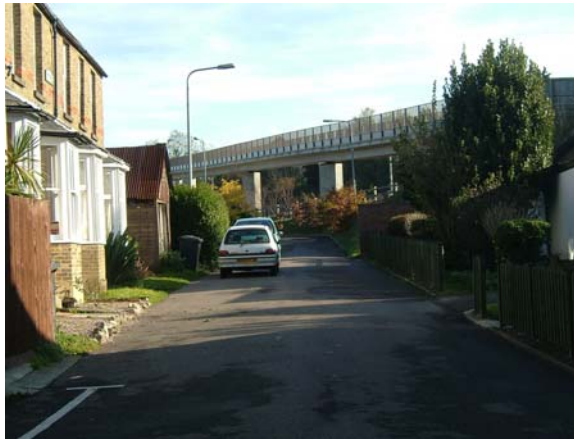
Pedestrian bridge at the end of Bowes Lane
