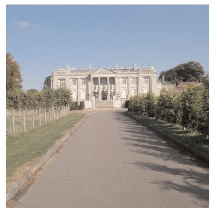
Approach to the House from the A2(T)
