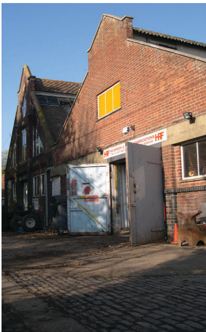
Farm buildings and architectural details within the main Highland Court model farm complex.
