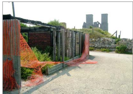
View of gateway into Conservation Area on eastern boundary
