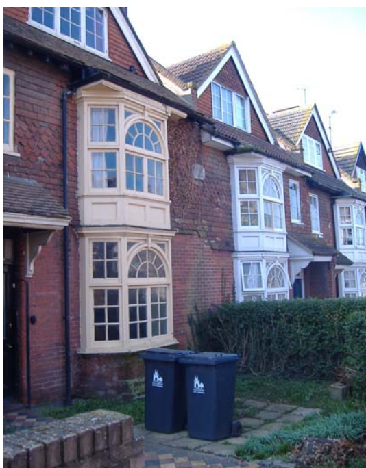
Tankerton Road – distinctive window design
