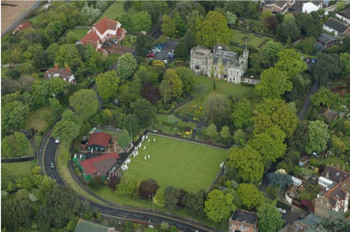
Aerial photograph of the castle, the grounds and setting
