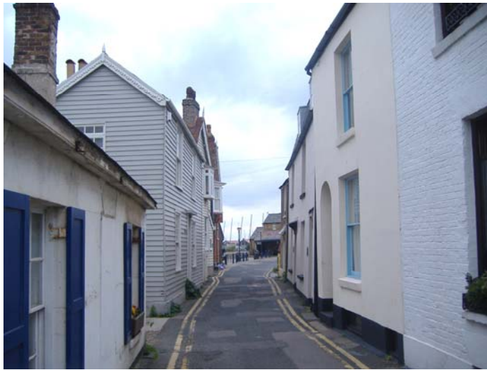
Sea Wall looking north
