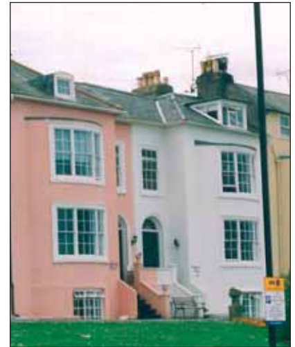
Unaltered pre-1840 houses, Marine Terrace
