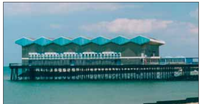
The present sports hall pavilion.
