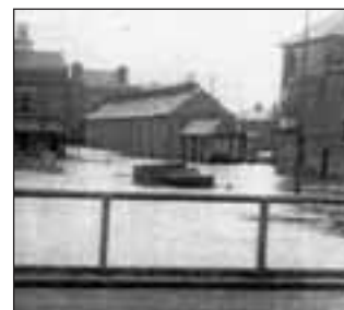
Flooding seen from High Street, 1897 (Gough)
