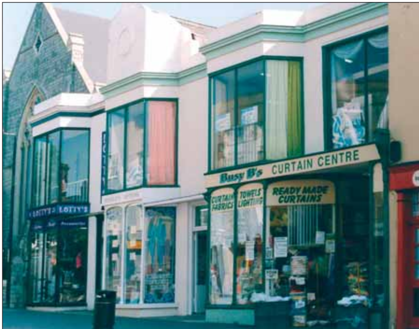
Mortimer Street two storey purpose built shop.
