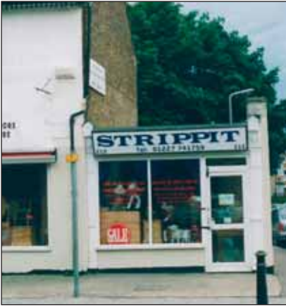
Single storey shop, High Street.
