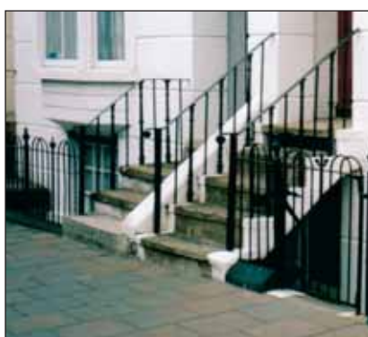
Original 19th century railings, Mortimer Street.
