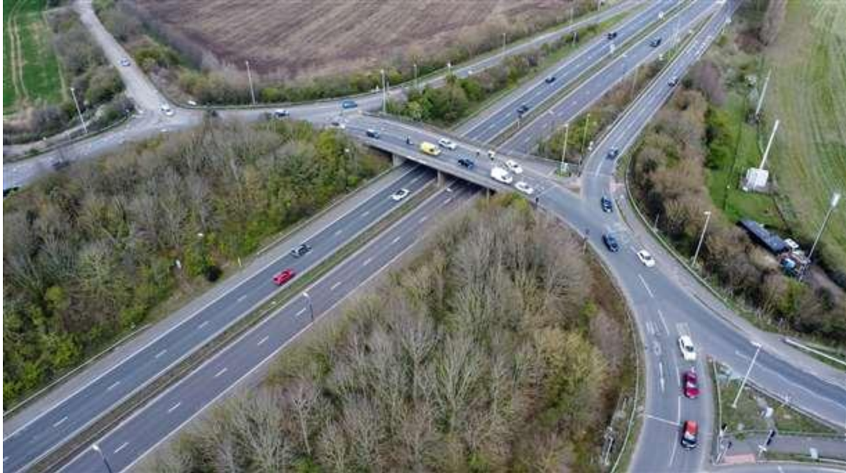
Brenley Corner will miss out on crucial government-funded upgrades. Picture: Barry Goodwin
