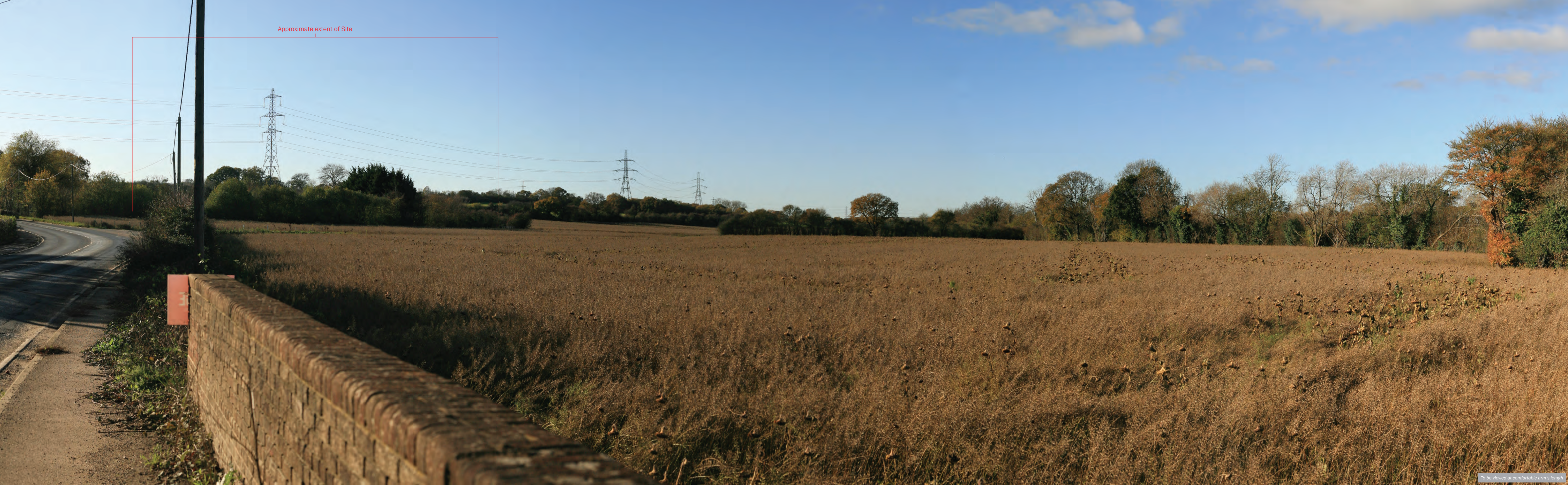
Photoviewpoint EDP 1: A291 (road) – Views for receptors looking south from footpath along A291 on Calcott Hill
