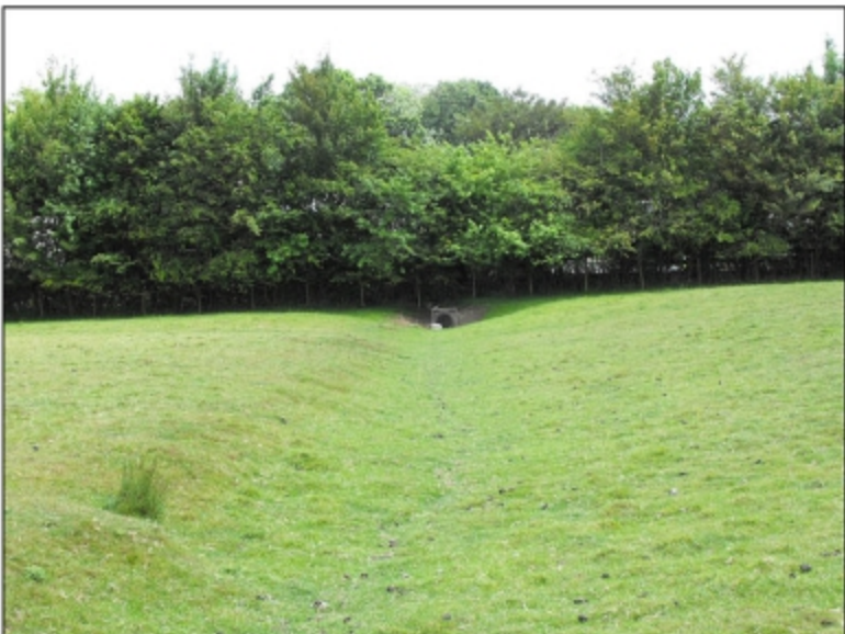
Plate 9. Gully with concrete drain. View facing south.
