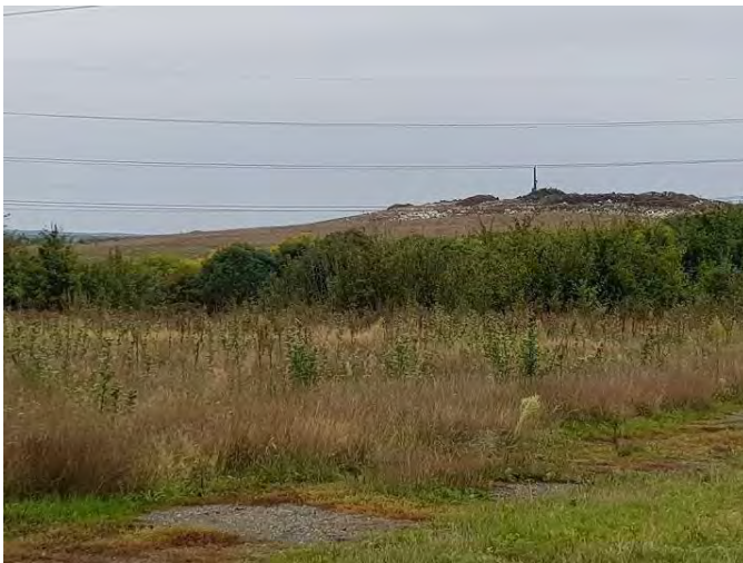
Shelford landfill and gas recovery
