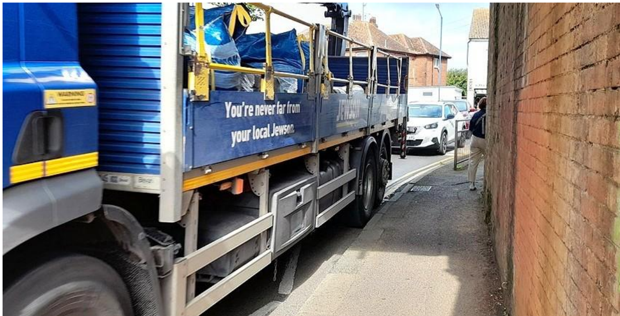
Figure 27: The narrow pavement under Chestfield railway bridge – suitable for children to walk both northwards and southwards to different schools at the same time?
