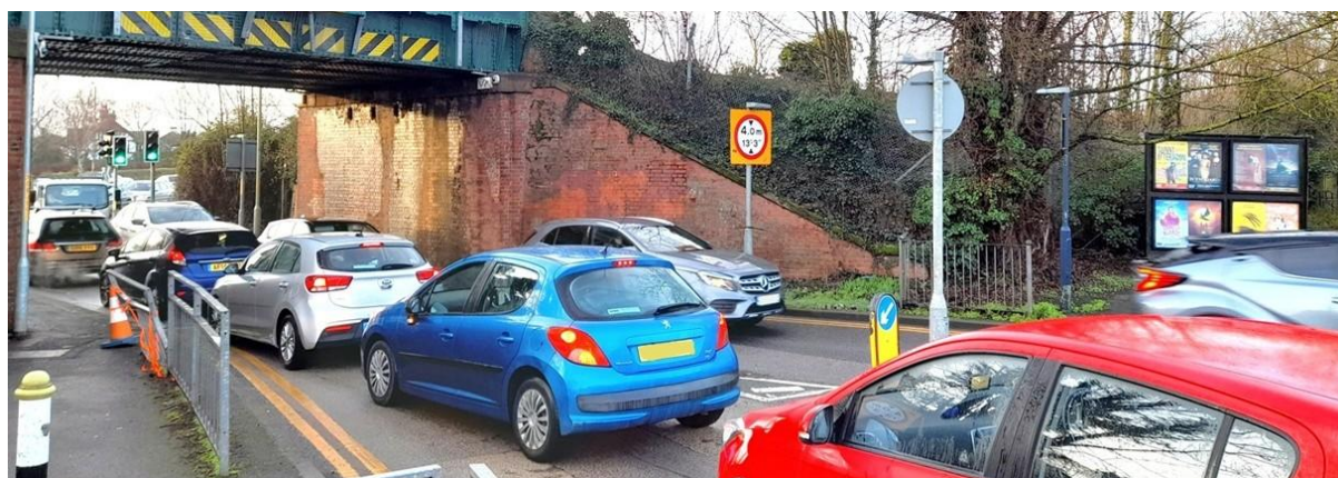
Figure 26: Traffic congestion at Chestfield railway bridge at 8.30am on a typical morning
