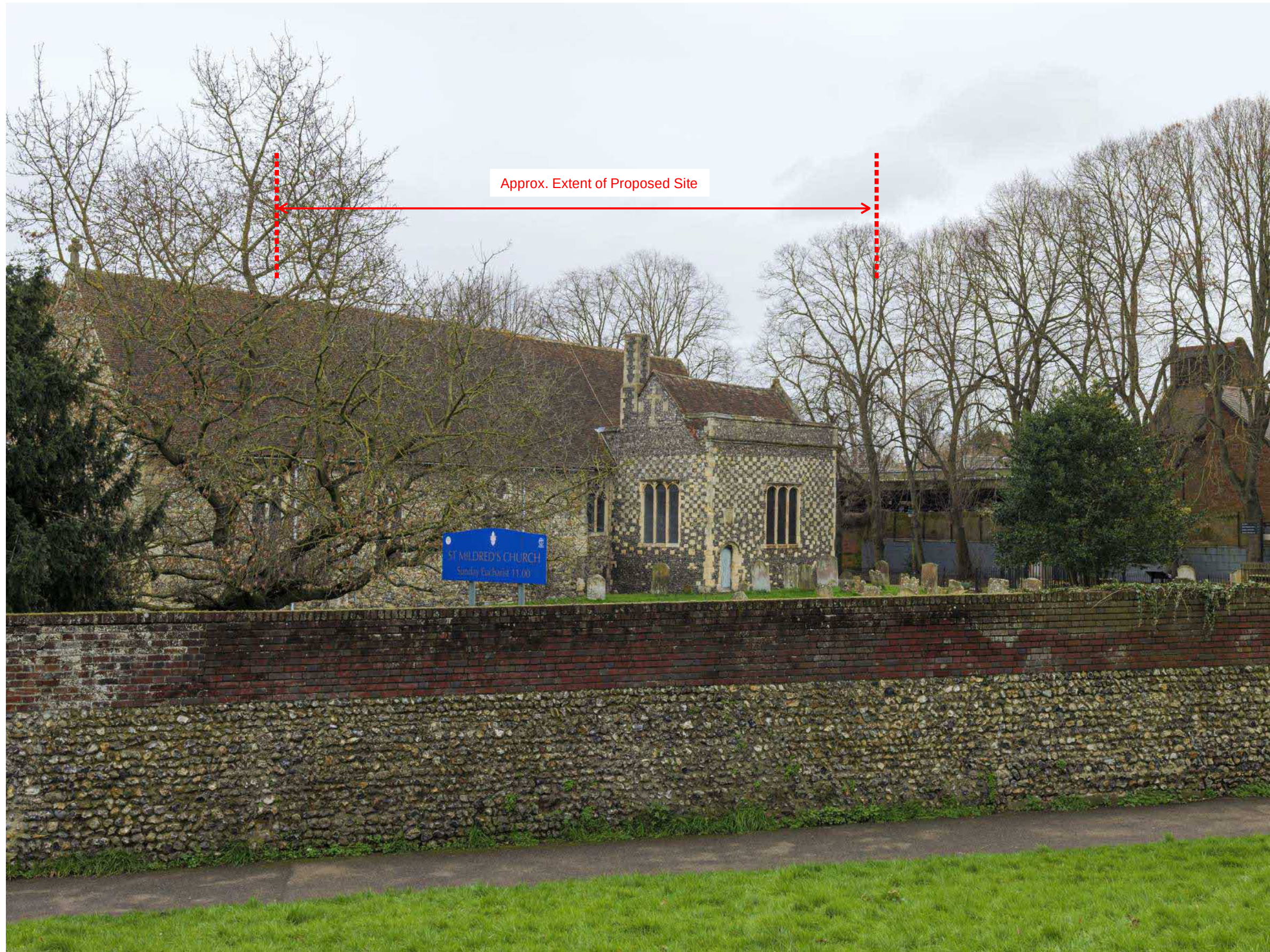
Fig. 104: Rosemary Lane 021 Site not visible (WINTER) © OSG Architecture Ltd
