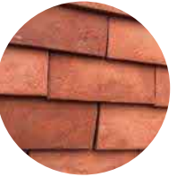
Tile hung cladding
