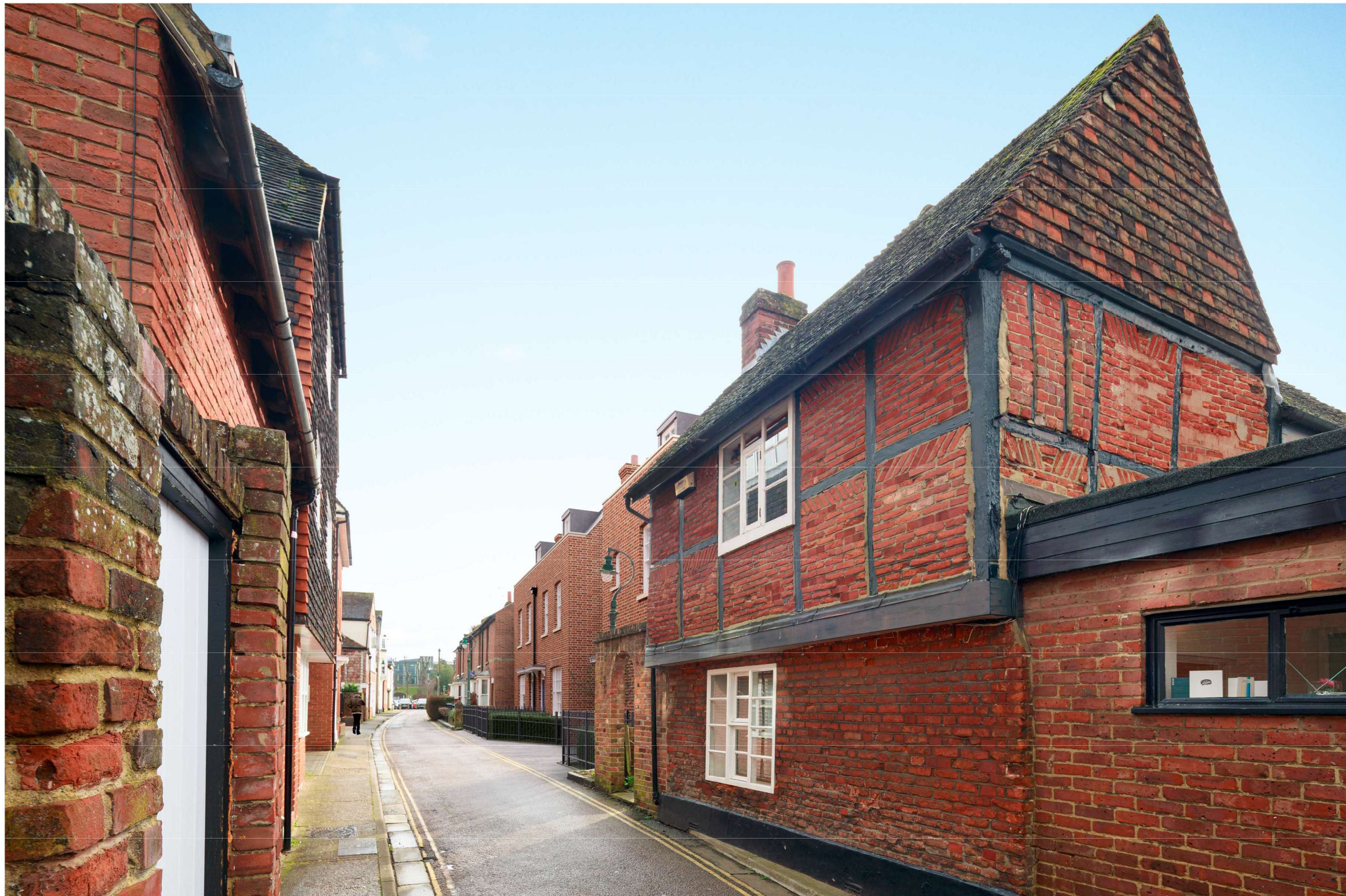
View southeast along St John's Lane
