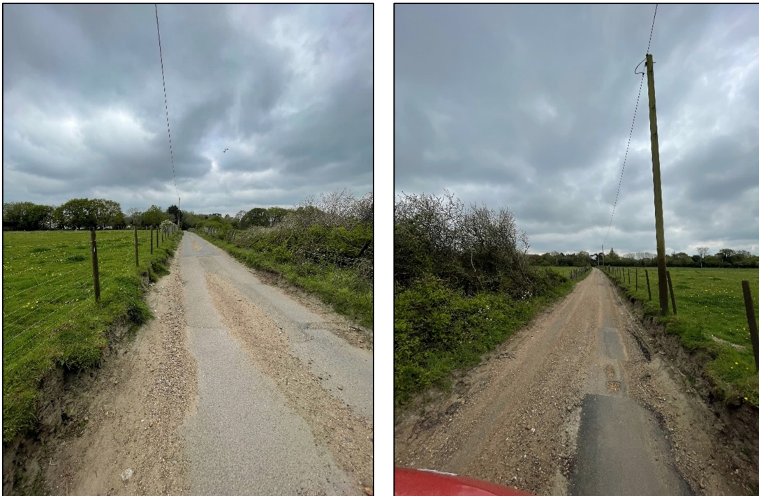
Figure 13 – Well Lane existing highway conditions
