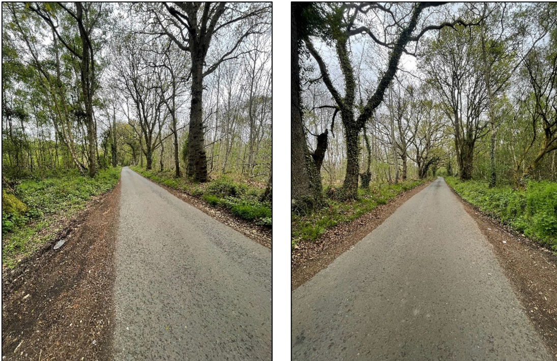
Figure 16 – Swanton Lane existing highway conditions
