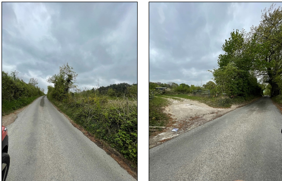
Figure 8 – New House Lane existing highway conditions
