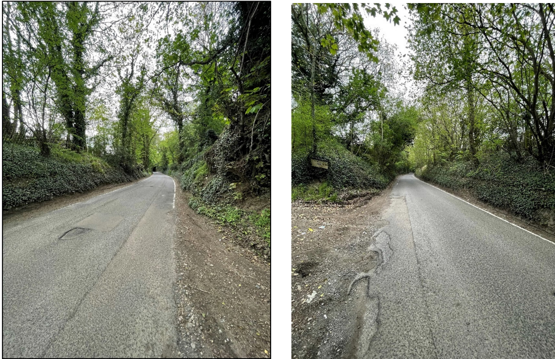
Figure 7 - Hollow Lane existing highway conditions
