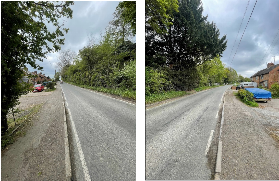
Figure 17 – Bekesbourne Lane (East) existing highway conditions
