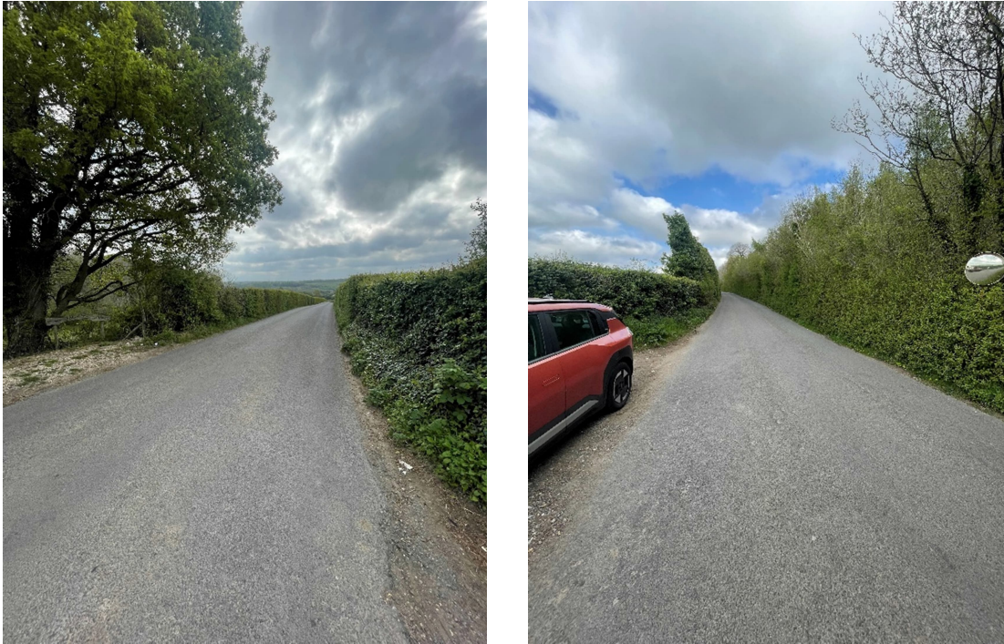
Figure 5 – Howfield Lane existing highway conditions
