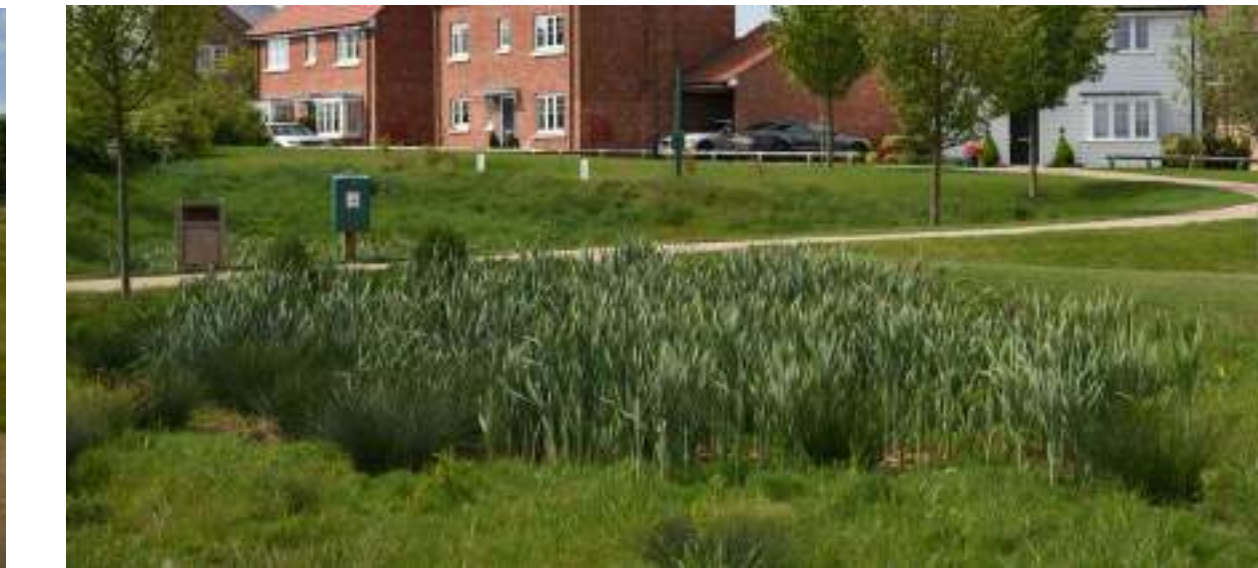
Dry landscaped attenuation basin
