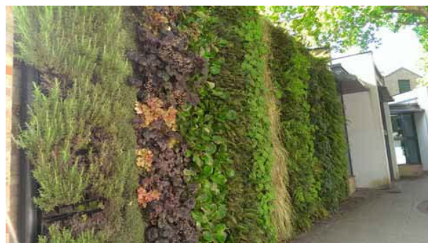
Plate 4.53 Living wall to Aphra Lumley Building
