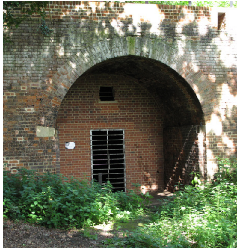
Grade II* Listed Tyler Hill Railway tunnel
