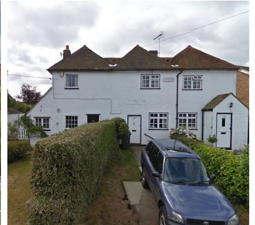
Grade II Listed Taylors Cottages
