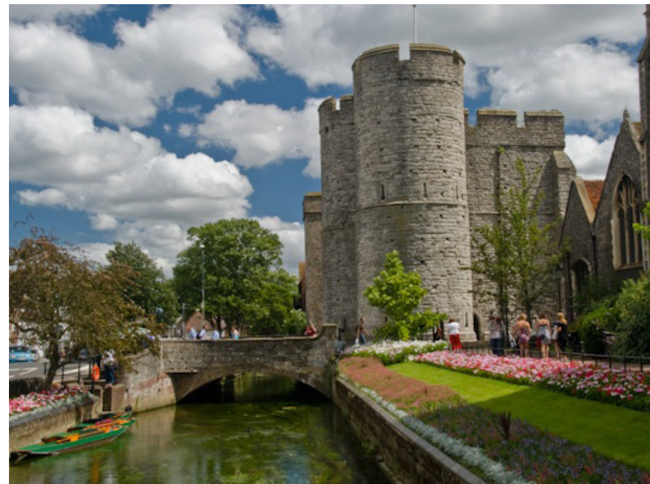
West Gate Tower, Canterbury
