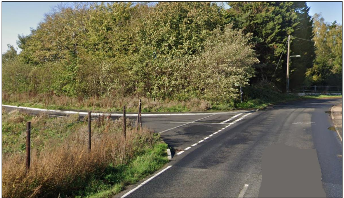
Figure 3.2: New access on Shalloak Road (Google Maps)
